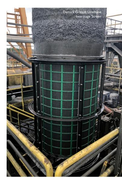
To date, many G-Vault screens have now been installed in multiple countries. Designed as a direct bolt-in replacement for the current wedge-wire interstage screens, the G-Vault is easily installed on site. Installation of the new technology, therefore, has little effect on operations, as changing screens is already a known procedure. In addition to improving operations, the G-Vault also benefits the operation's workforce, as it makes room to reallocate resources.
