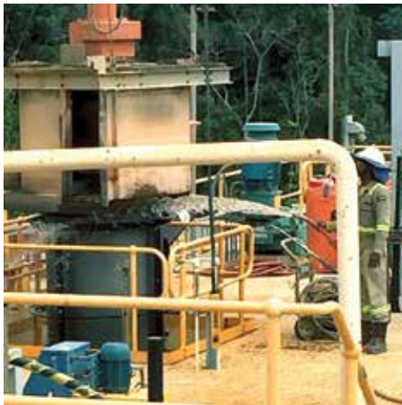
Figure 1 - washing of interstage screen at CIL plant
