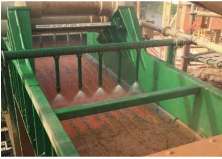
Derrick vibratory screening machine upgrade in place of existing equipment
