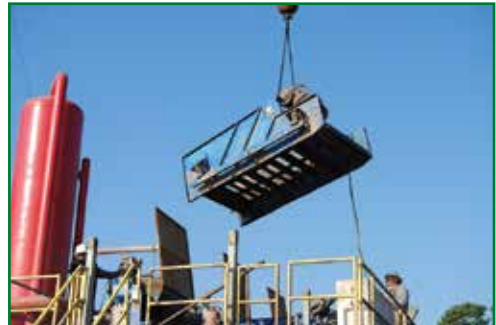
Remove basket and pivot frame.
